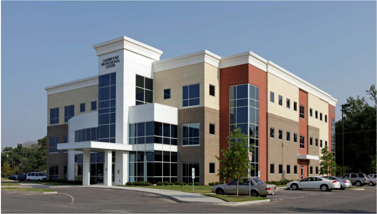
Facing Front; South Side
