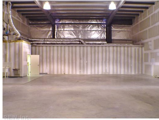
REIN, Inc. Warehouse
