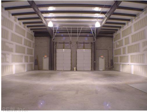
REIN, Inc. Warehouse
